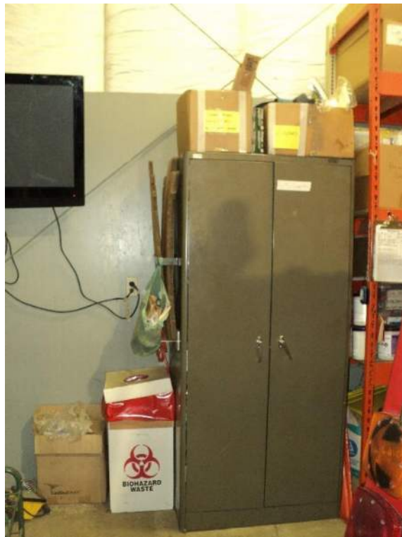
Image 7: Tall and Narrow Unbraced Storage
