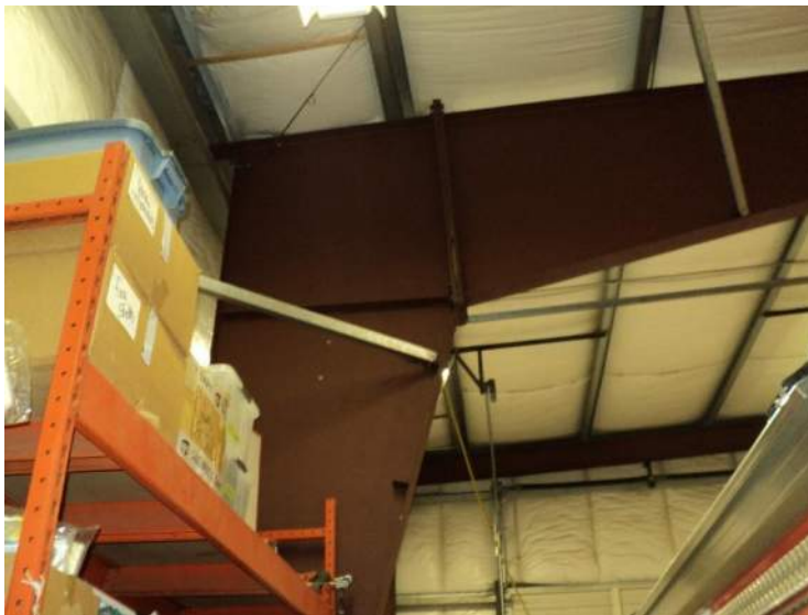
Image 6: Existing Steel Moment Connection
